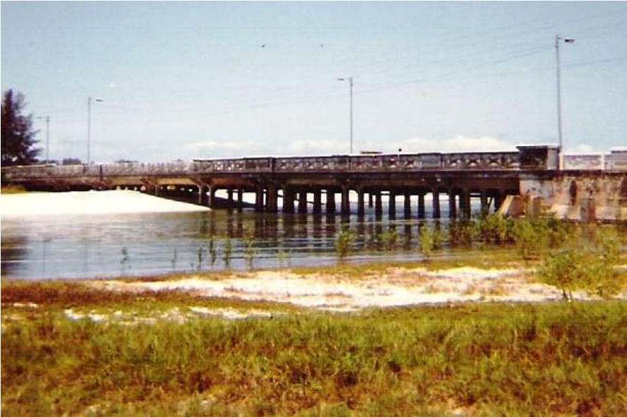
Selander Bridge in Dar. On the right is the Indian Ocean.
